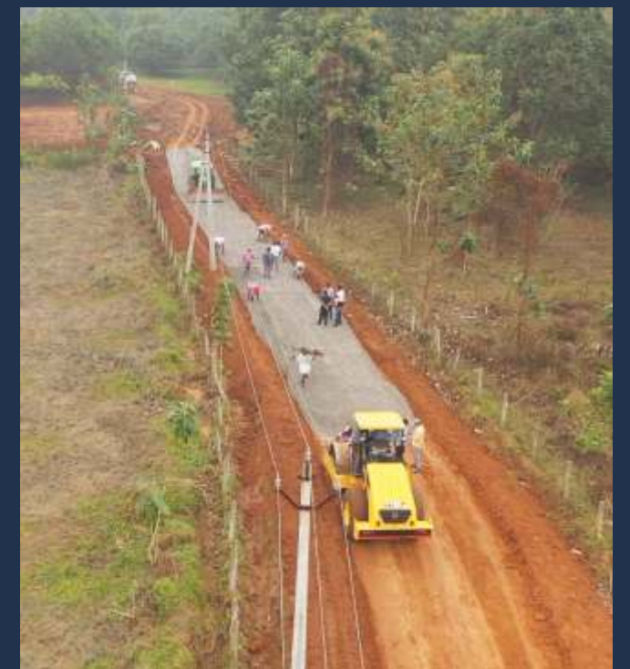
(Actual Photograph from site)
